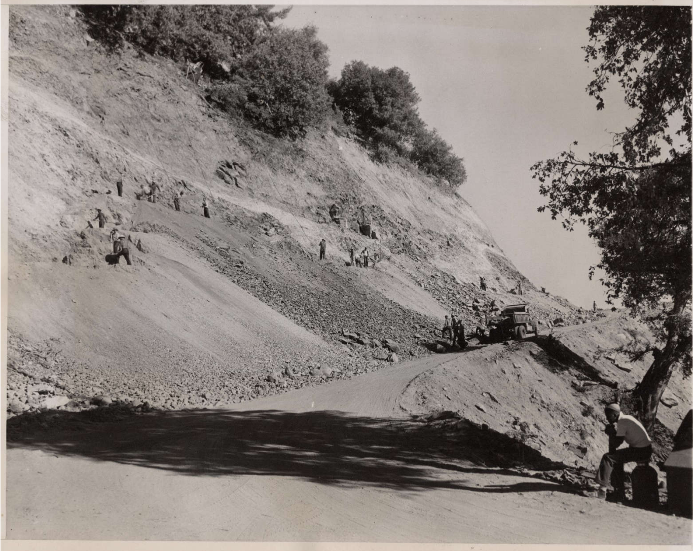
LA 418669 "MOVE MOUNTAINS" IN BUILDING MT. PALOMAR OBSERVATORY WORKMEN CHANGING THE ESCARPMENT OF PALOMAR MOUNTAIN, NEAR SAN DIEGO, CALIF., WHERE SCIENTISTS ARE SUPER- VISING CONSTRUCTION OF A $6,000,000 OBSERVATORY TO HOUSE THE 200-INCH "EYE"--WORLD'S LARGEST TELE- SCOPE. THIS WORK WILL PREVENT EROSION OF THE MILLION DOLLAR HIGHWAY BEING BUILT UP THE SIDE OF MT. PALOMAR TO THE OBSERVATORY, WHICH WILL BE COMMISSIONED IN 1939. (#1B FOR JAP AUS) CREDIT LINE(ACME) 11/9/37
