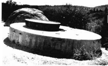
"Concrete eye" which doubled for the famous 200-inch mirror during construction
